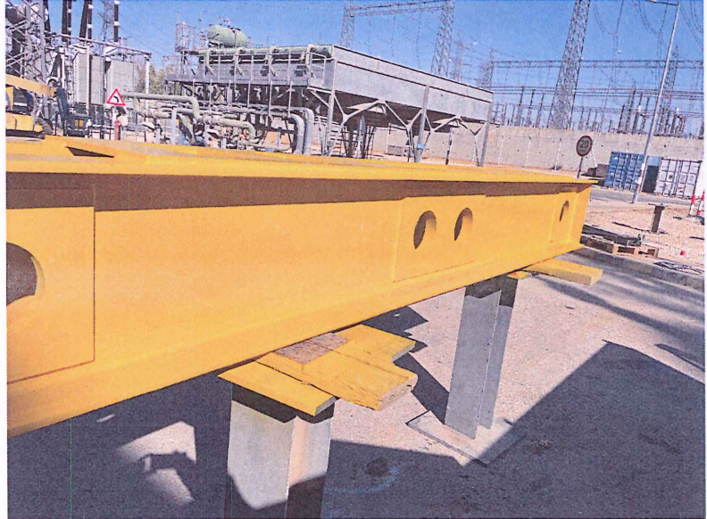
Final paint layer combustion Chamber lifting Device
