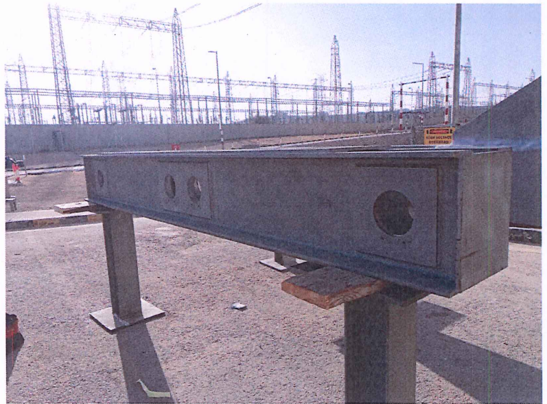
Combustion Chamber lifting beam after sand blasting
